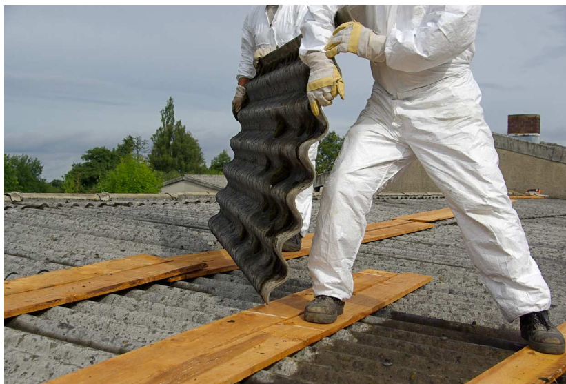
Removing asbestos
